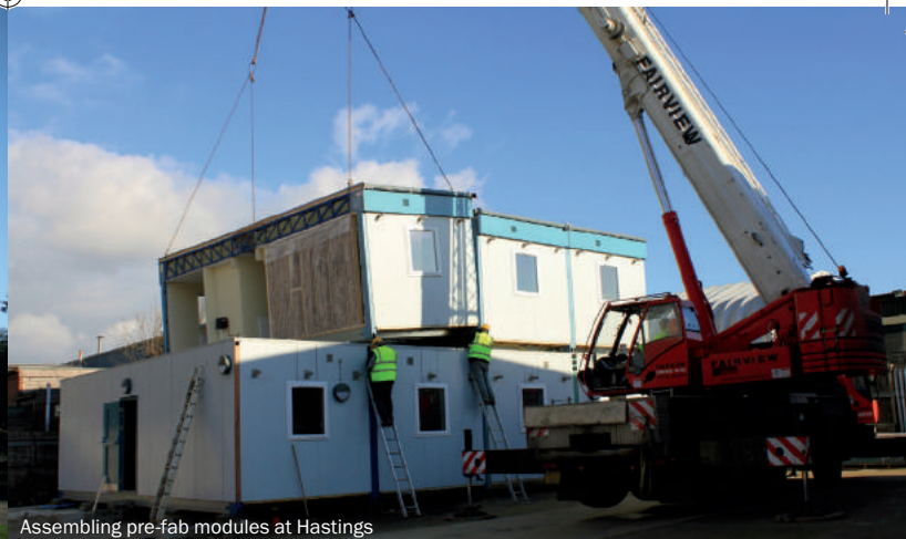
Assembling pre-fab modules at Hastings
